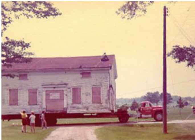
Heritage House on its way to Silver Springs Park, photo circa early 1970's
